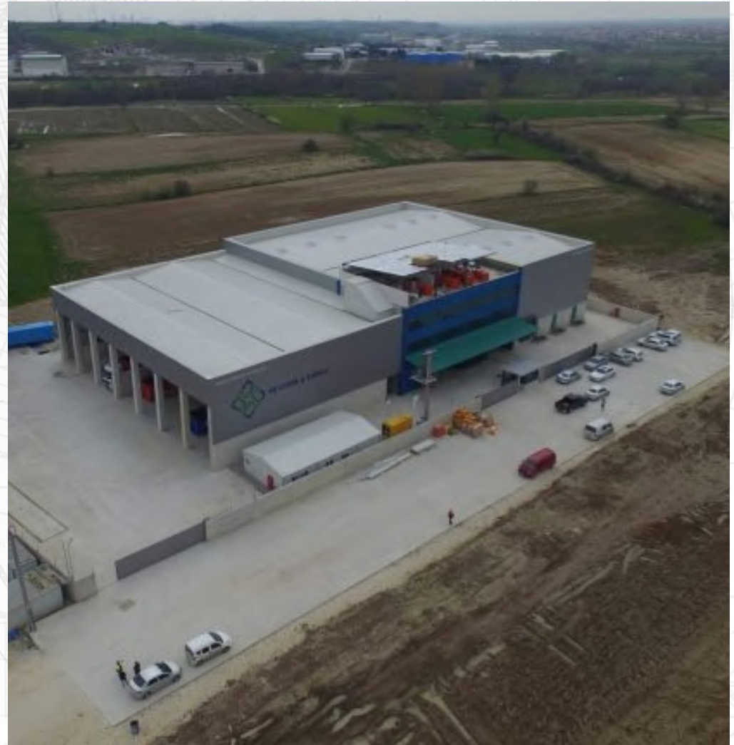
Structural System Concrete and steel construction
