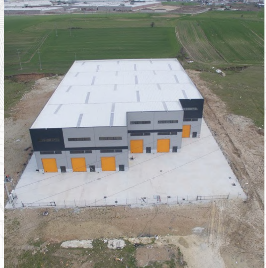
Structural System Precast Construction
