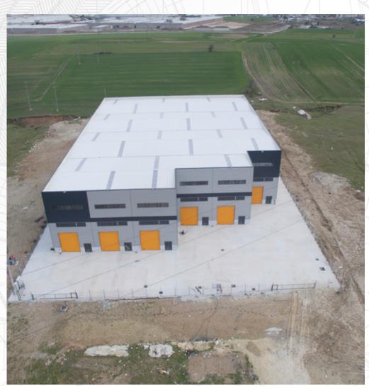
**Structural System**Precast Construction
