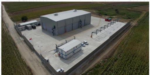
**Structural System**Precast and conventional concrete and steel construction
